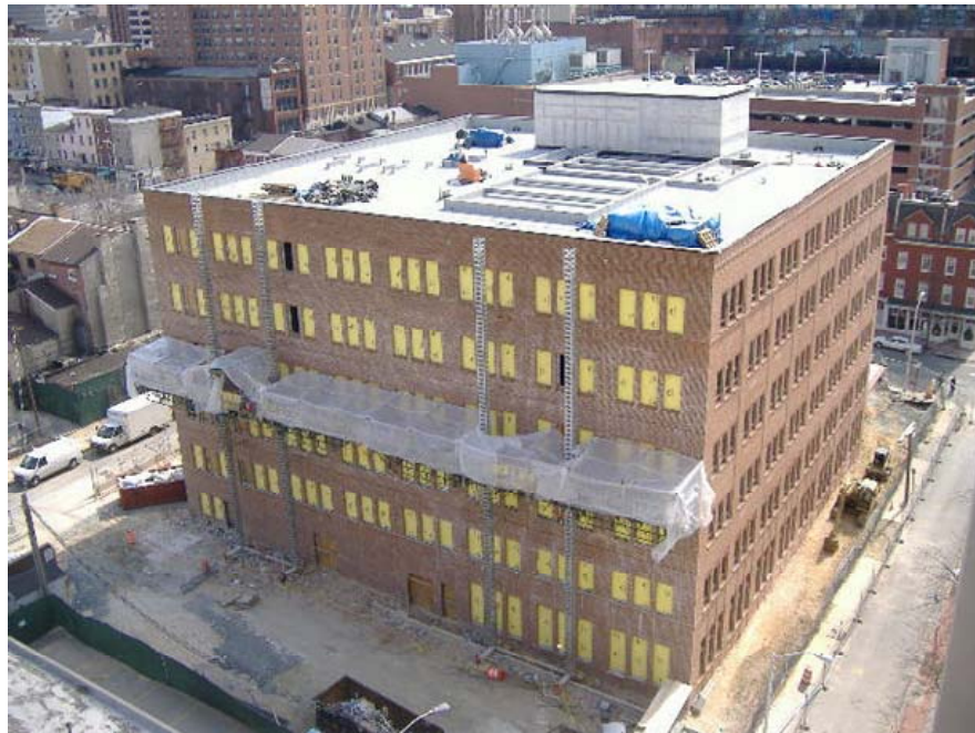
Figure 5b Façade Scaffolding.
