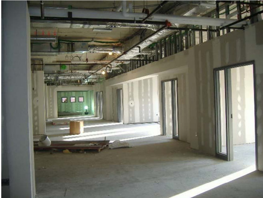
Figure 4 Drywall and mechanical installation.
