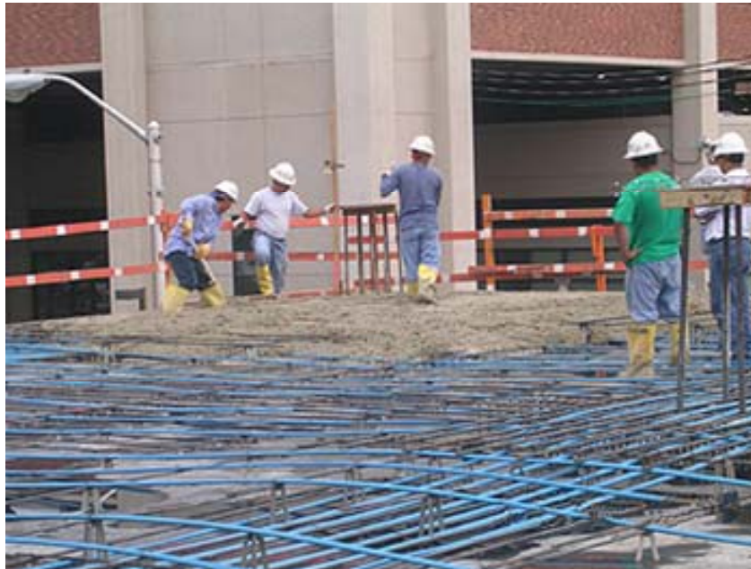
Figure 3 Reinforcing at interior column.
