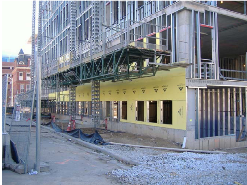
Figure 5a Façade scaffolding.
