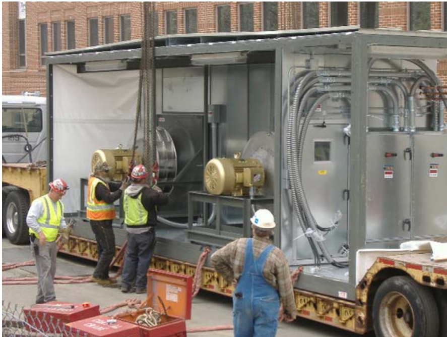
Figure 6 1 of 8 AHU Components delivered on site.
