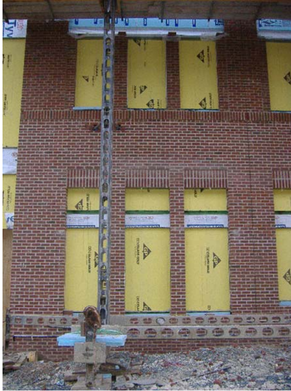
Figure 3 Brick window detail.
